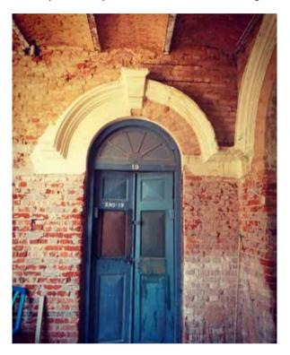
some of its walls. Right now, deteriorated plasterwork is being reworked using lime mortar which is prepared on site. The reapers of the first floor roof are being inspected and replaced or repainted as necessary. Cornice and arch moulding are also being repaired and reconstructed.
